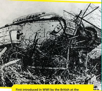
Battle of the Somme in 1916, tanks could easily roll over barbed wire, allowing soldiers to cross "No Man's Land" between the trenches. Machine guns and cannons were mounted on tanks to deflect attack from enemy soldiers. However, early tanks often got stuck in the mud, and because they moved slowly, were vulnerable to machine-gun attack. Q: Did the British decision to introduce tanks fairly consider the needs of the British soldiers?
